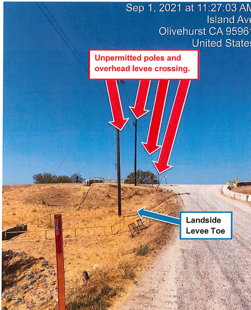
Photo 6: View of Unpermitted PG&E power poles and overhead utility line crossing the levee.
